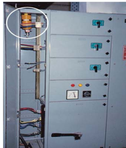
typical vertical model installation inside electronic panel
