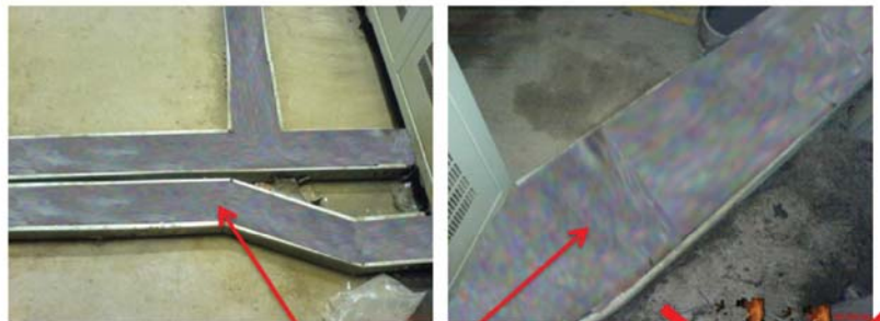
cable trench filled with nasa flame retardant chemical granules
