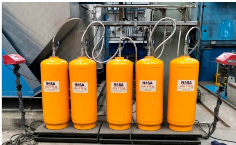
Typical NASA fire suppression system installation
